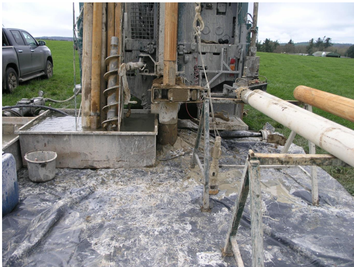
Figure 18: Bore-hole drilling north of the Campile River
