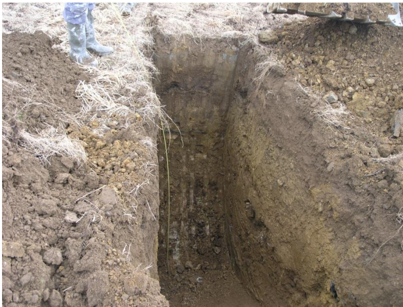
Figure 17: Baginbun Test Pit TP02-1
